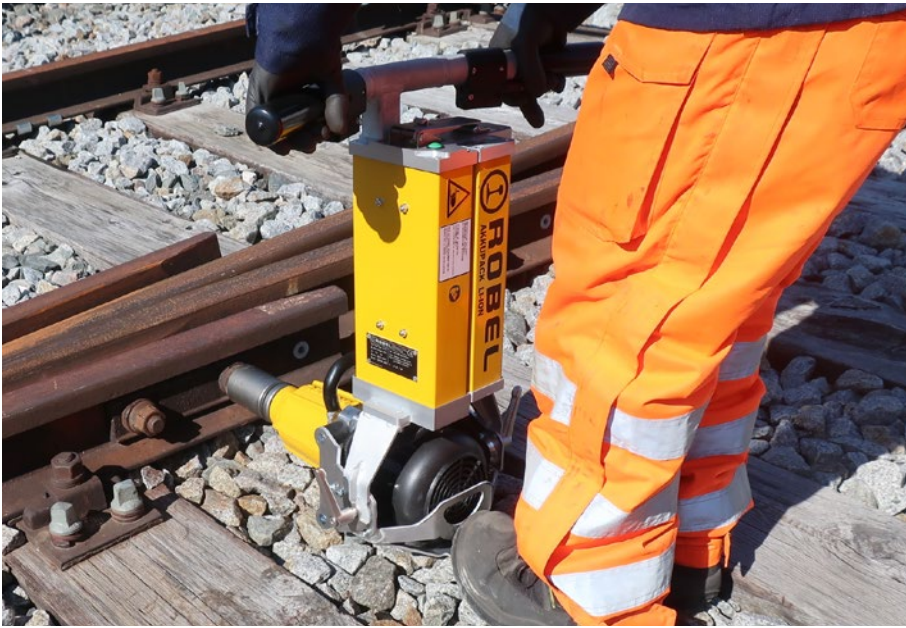
Fig. 6: Power wrench 30.20 E3 can be adjusted for horizontal or vertical work
